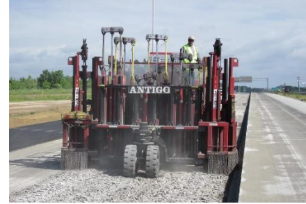
Rubblizing - Photo courtesy of Antigo Construction
