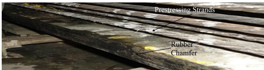
Figure 4.3. Precasting bed with removable rubber chamfer
