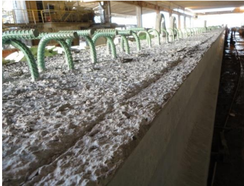
Figure 4.16. Inconsistent troweled surface along the length of the PPCB
