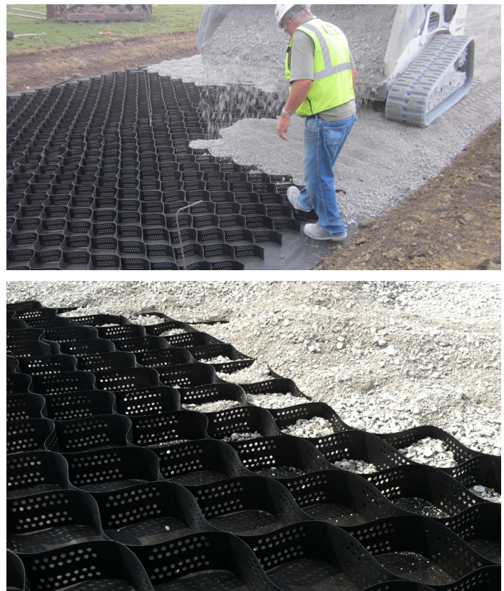
Figure 2. Placement of crushed limestone base in 4 in. geocells
