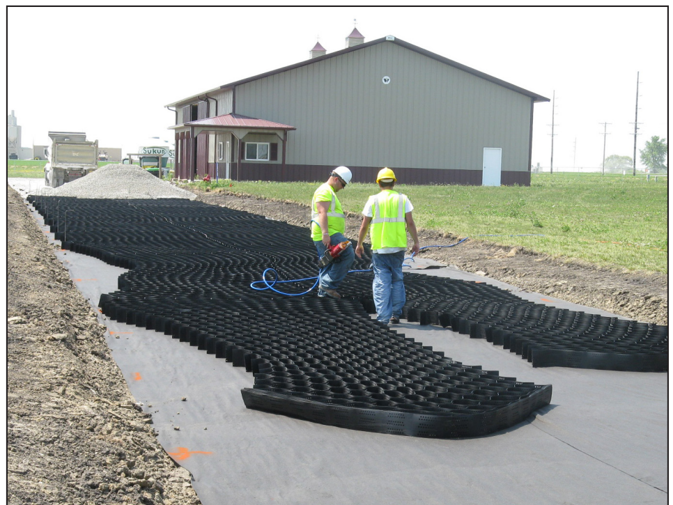
Figure 1. Installation of 6 in. geocells over non-woven geotextile placed on subgrade
