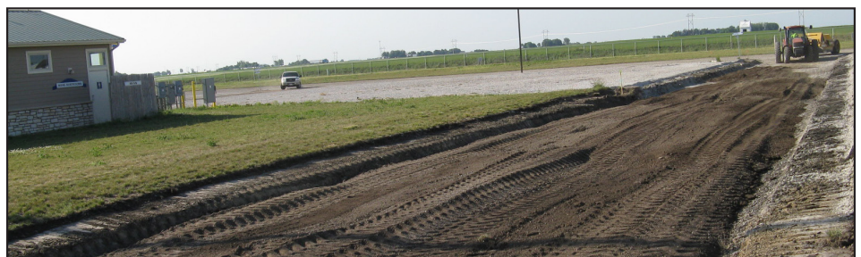
Figure 1. Reclaimed subbase material placed on 9th St. North
