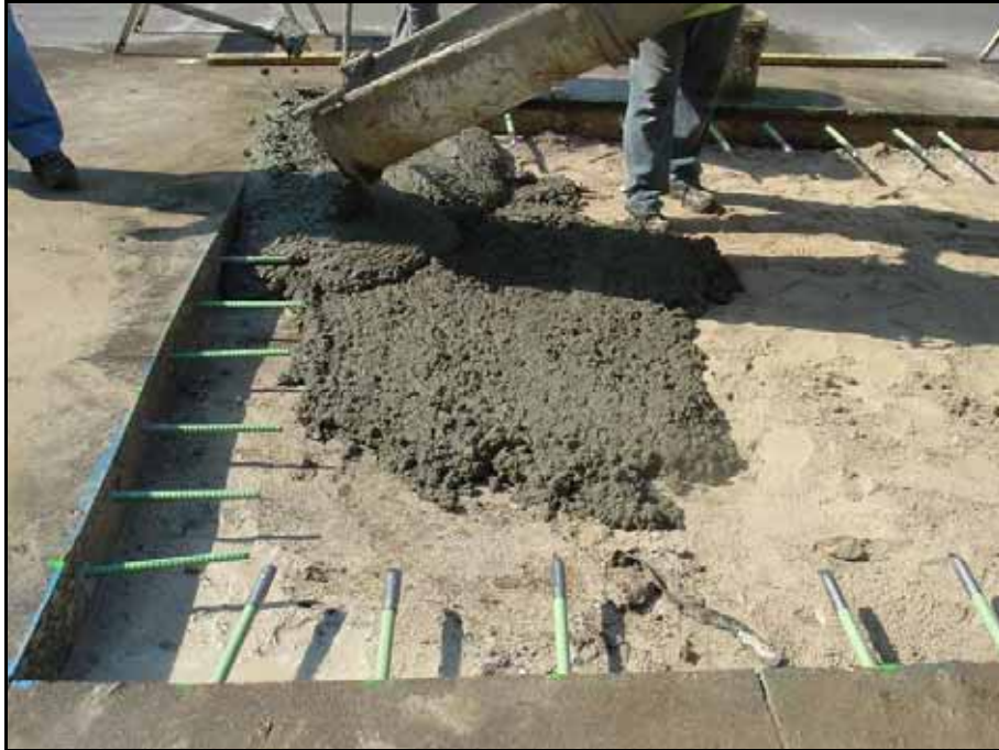
Figure 49. Concrete placement in Des Moines
