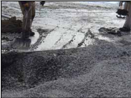
(a) Cleaning excess material into the trench
