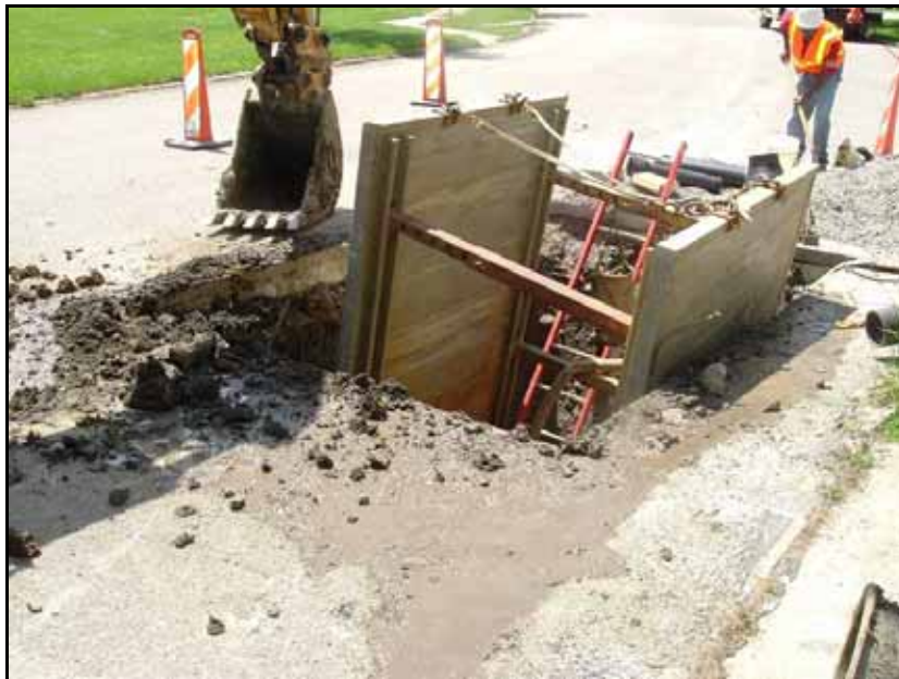
Figure 40. Shoring box in place
