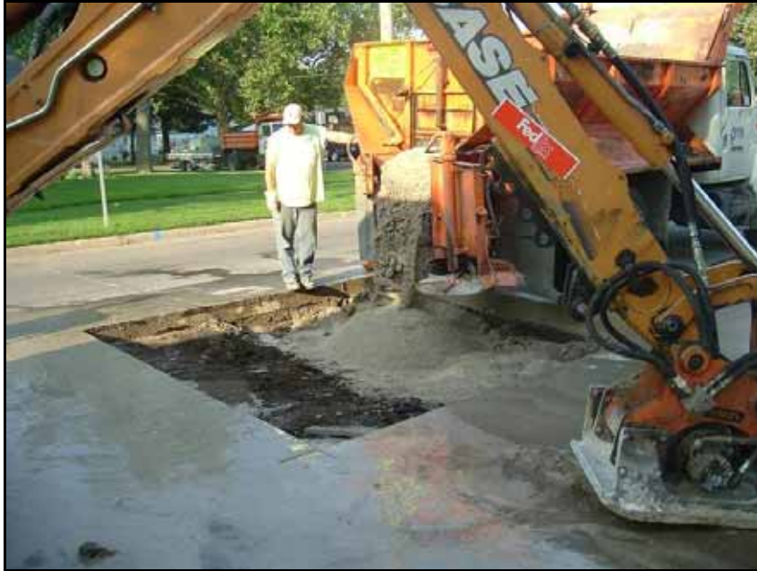
Figure 47. Adding additional manmade sand to the trench
