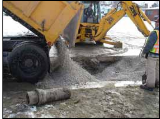
(b) Dumping backfill material
