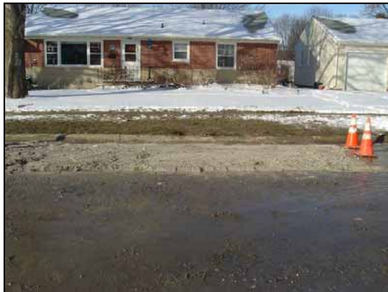
Figure 39. Trench ready for cold patch
