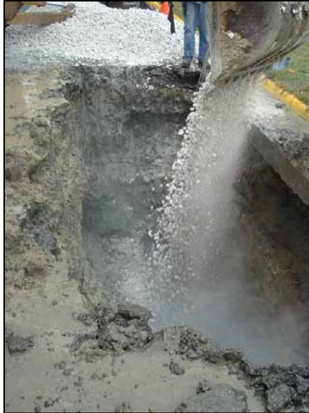
Figure 27. Bedding material dumped into trench
