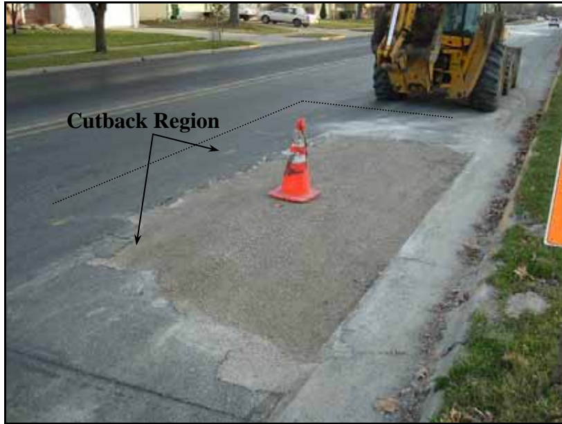
Figure 57. Site in Ames two weeks after construction
