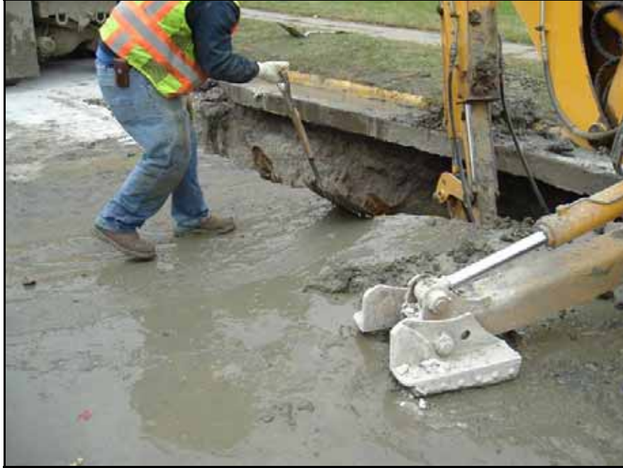
Figure 29. Saturated material shoveled into the trench
