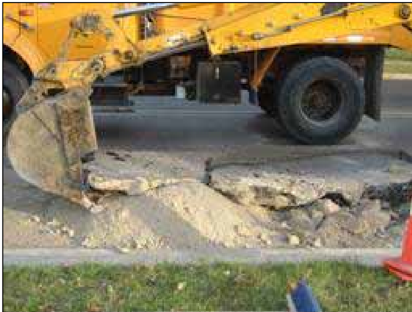
Figure 58. Pavement removal
