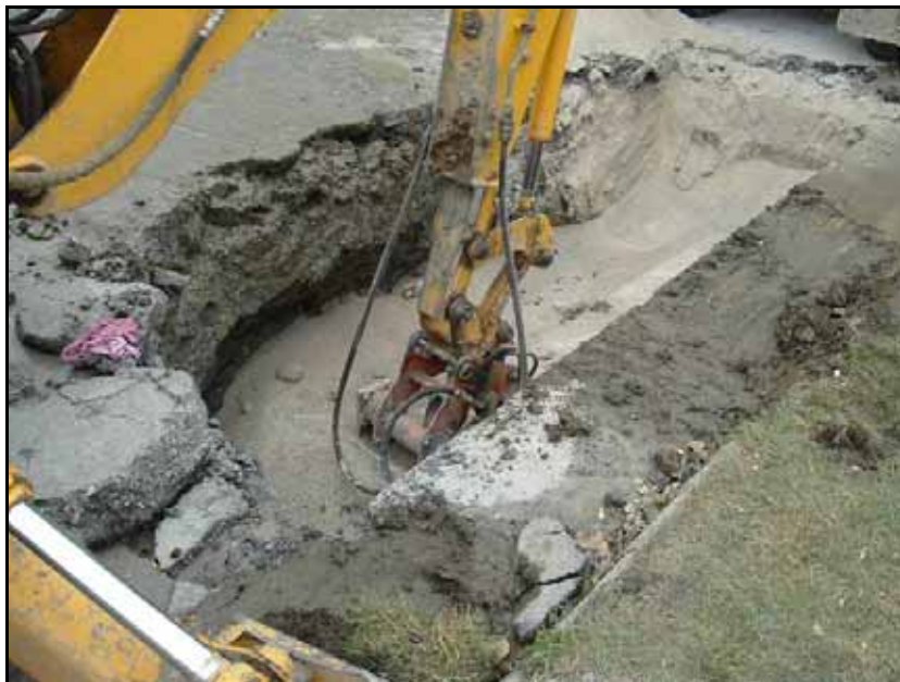
Figure 28. Compaction of backfill material
