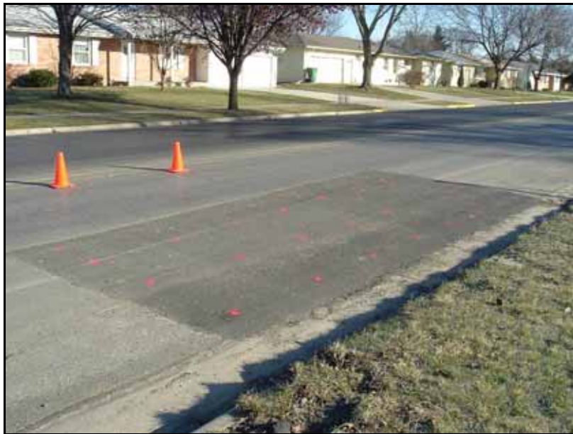
Figure 33. Ames site completed
