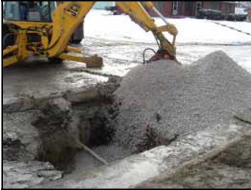
(a) Pushing in backfill material
