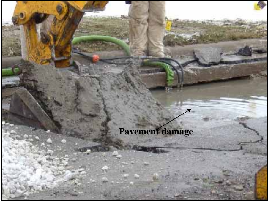
Figure 36. Saturated material being excavated
