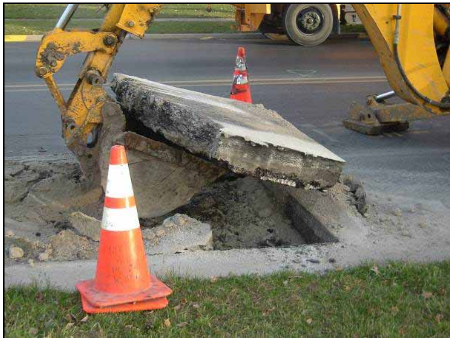
Figure 31. Pavement removal
