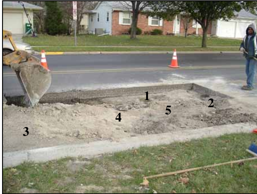
Figure 59. Testing layout of trench
