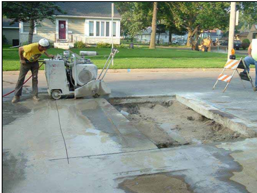
Figure 46. Concrete pavement cut being made
