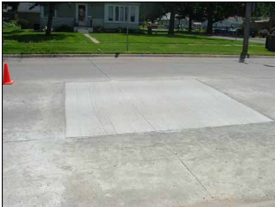
Figure 50. Completed surface in Des Moines
