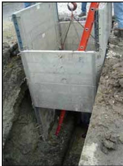
Figure 26. Shoring box placed into trench
