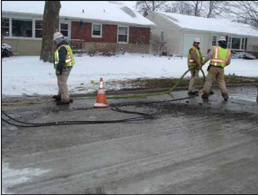
Figure 35. Dewatering the trench
