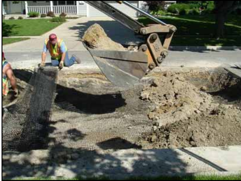
Figure 94. Geogrid being placed
