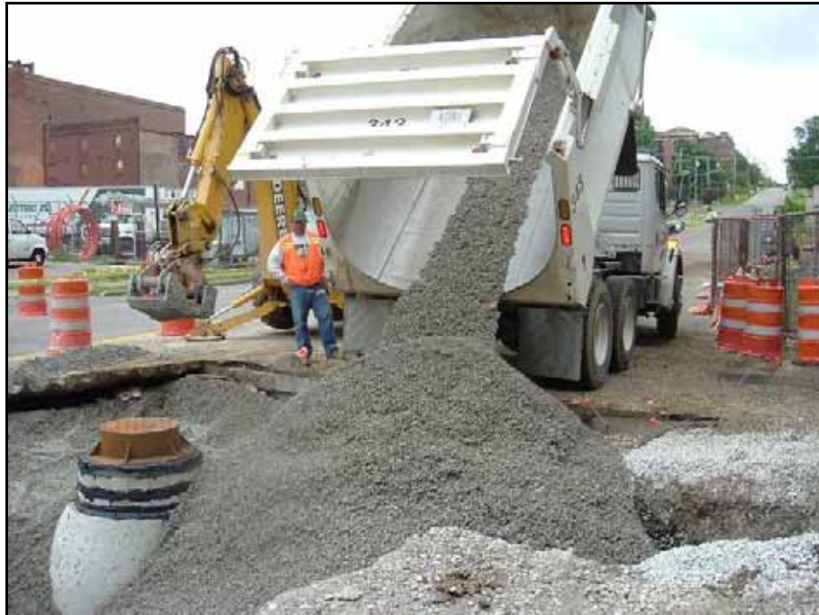
Figure 43. Large backfill lift being placed
