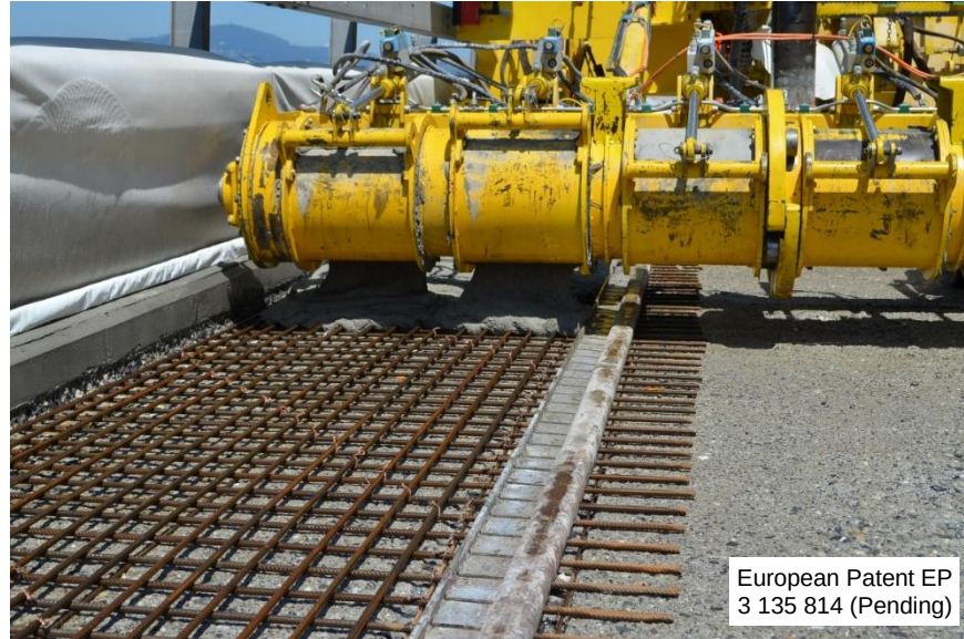
Figure 2.4. Casting of UHPC during bridge deck strengthening on the Chillon Viaducts
