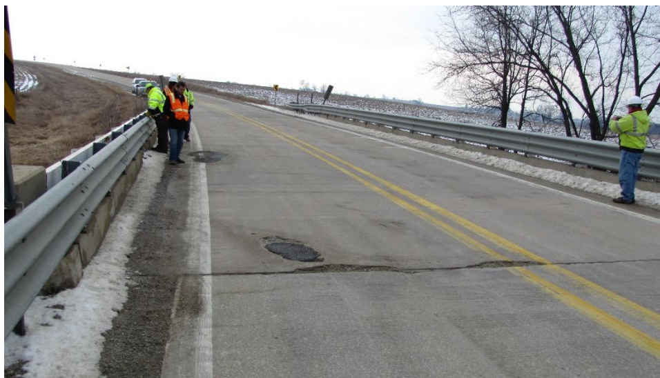
Figure 3.1. Mud Creek Bridge deck before UHPC overlay application
