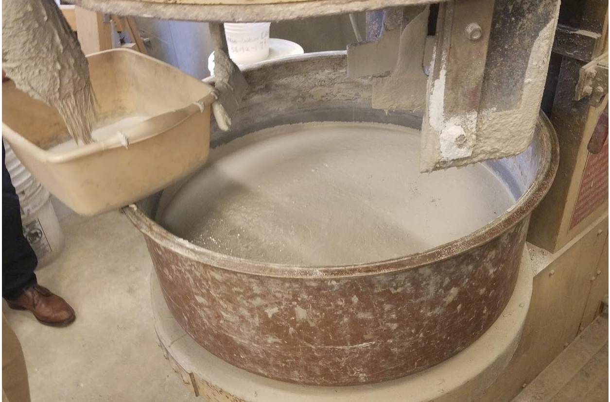
Figure A7. Demonstration of UHPC mixing
