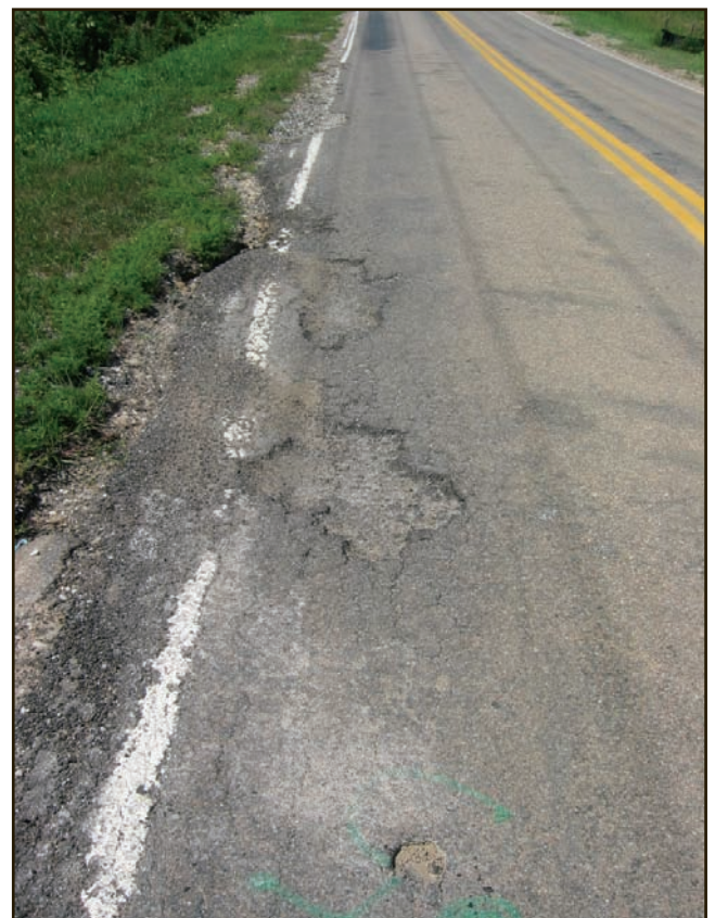
Figure 20. High severity rated potholes are 1–2+ inches deep and range from 18–30 inches in diameter.
