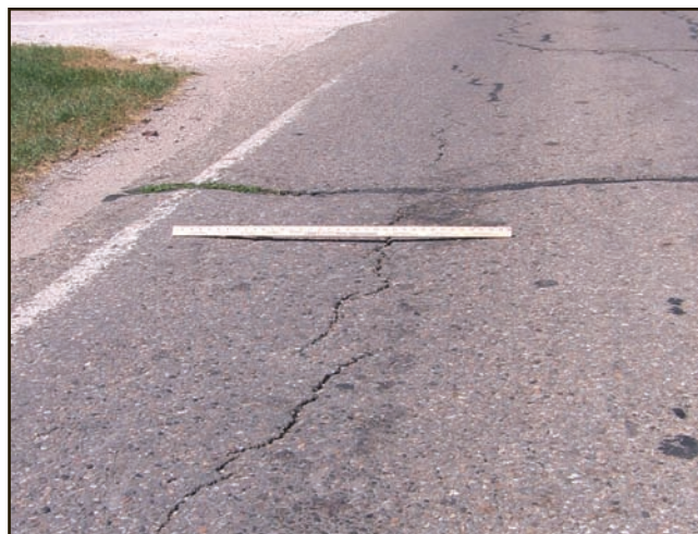
Figure 21. Longitudinal cracks at the bottom of rutting are often caused by structural failure of the subbase.
