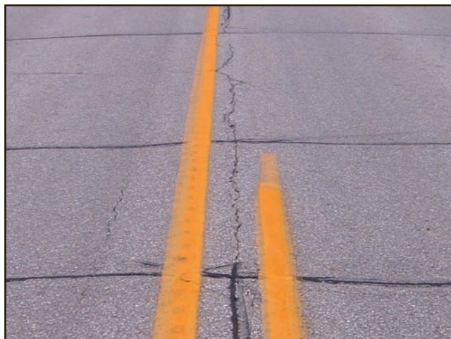
Figure 11. Longitudinal cracking can occur down the centerline where construction joints intersect, parallel to the direction of traffic.
