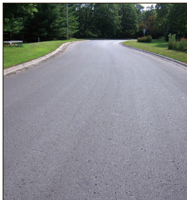
Figure 3. Light oxidation or pocking is a type of distress that makes a good candidate for a water-proof seal.
