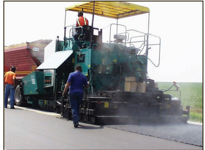
Figure 34. NovaChip® application.
