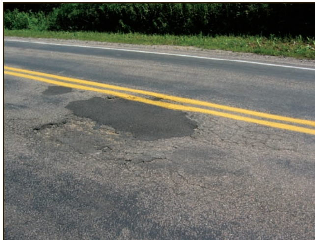
Figure 16. Medium ratings of patching are areas moderately deteriorated that had been replaced with new material.
