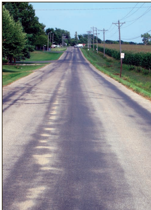
Figure 5. Low levels of bleeding are often the result of too much asphalt binder being pushed to the surface, but aggregate is still exposed, and asphalt does not stick.
