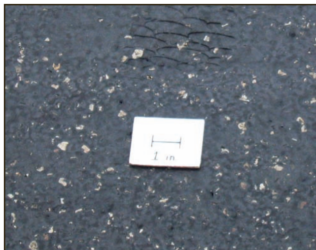
Figure 6. In high ratings of bleeding on pavements, shoes and tires stick to the surface and aggregate is barely visible.
