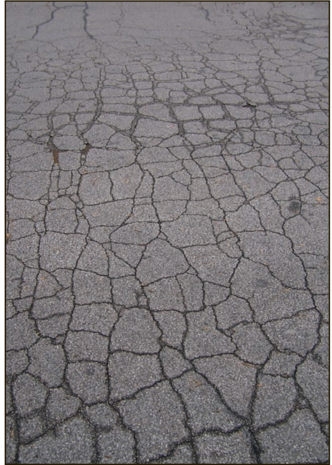
Figure 4. Alligator cracking is a distress that can sometimes be slowed by using a TMS as a stopgap, depending the level of severity and volume of traffic.
