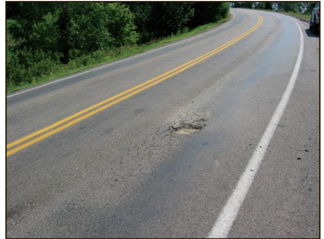
Figure 19. Potholes are a bowl-shaped hole in the pavement surface generally surrounded by alligator cracking.
