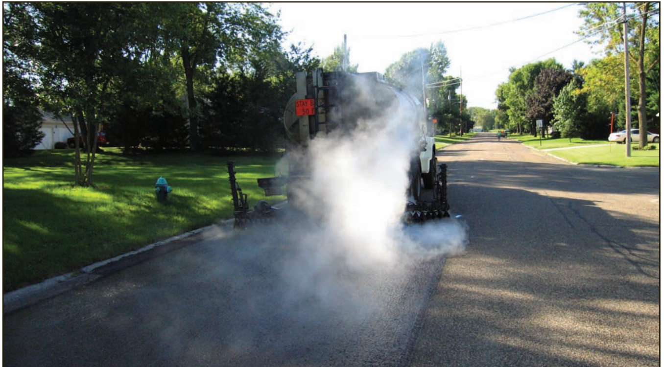
Figure 31. Fog seal application
