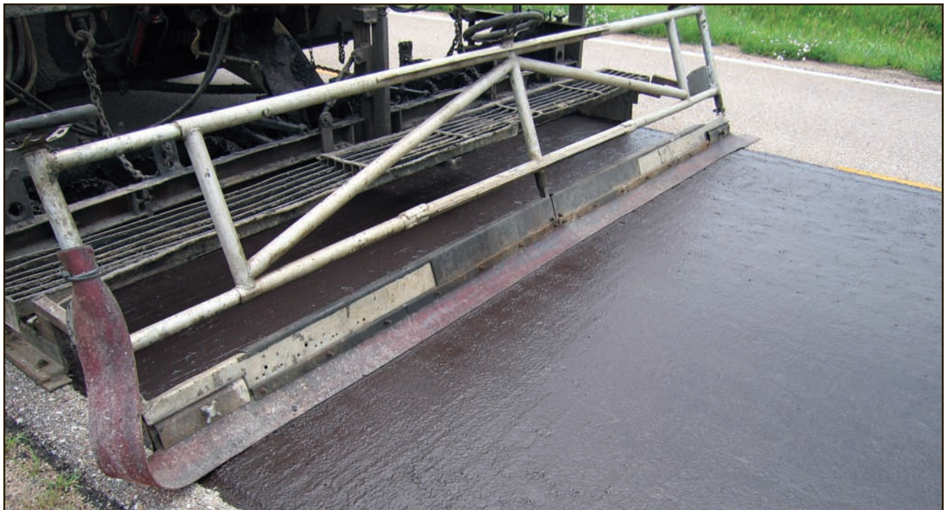
Figure 29. Slurry seal application.
