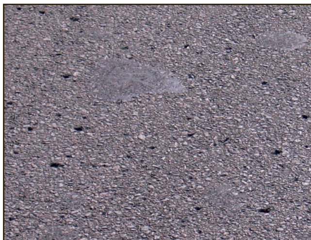
Figure 17. Pocking occurs when pieces of aggregate become dislodge or deteriorate prematurely.
