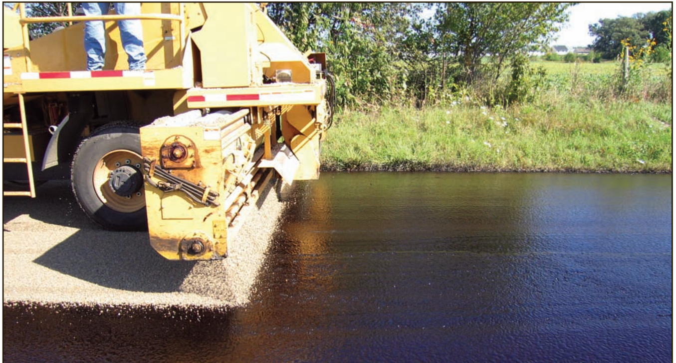
Figure 27. Seal coat surface treatment.
