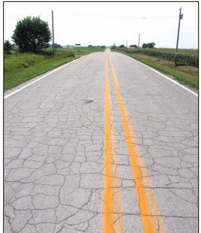
Figure 9. High block cracking ratings are those with cracks wider than \frac{3}{4} inch that are spalling. They occur over in large rectangles over the entire pavement.
