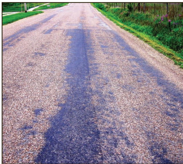
Figure 26. New raveling of a pavement surface.
