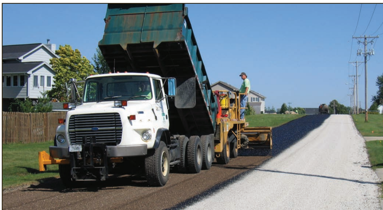
Figure 28. Double seal coat surface treatment.
