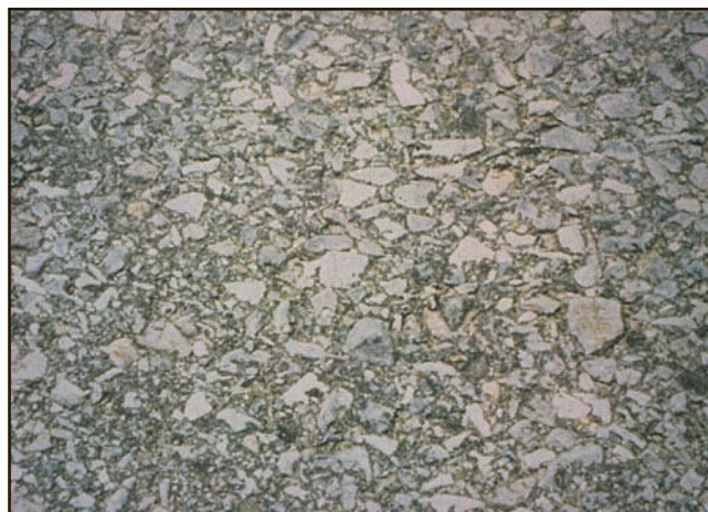
Figure 18. Polished aggregate is smooth pavement with little or no friction. (FHWA)
