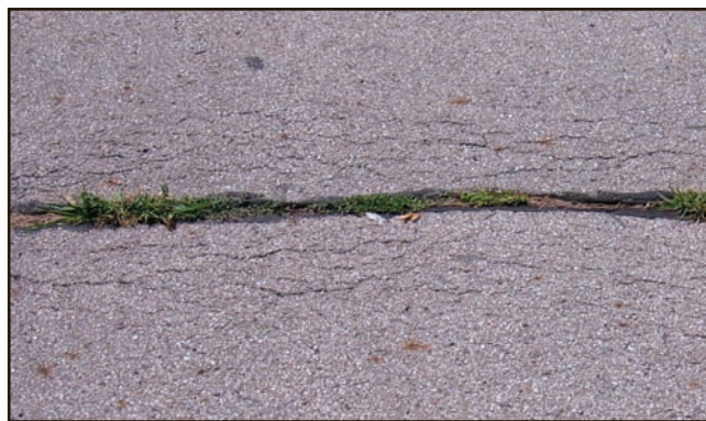
Figure 24. Low level spalling where parallel satellite cracks are beginning to form.
