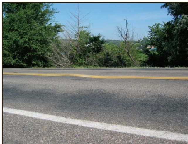
Figure 23. Shoving or corrugation of pavement surface is a longitudinal wave or bump in the asphalt, usually on hills, curves, or intersections.
