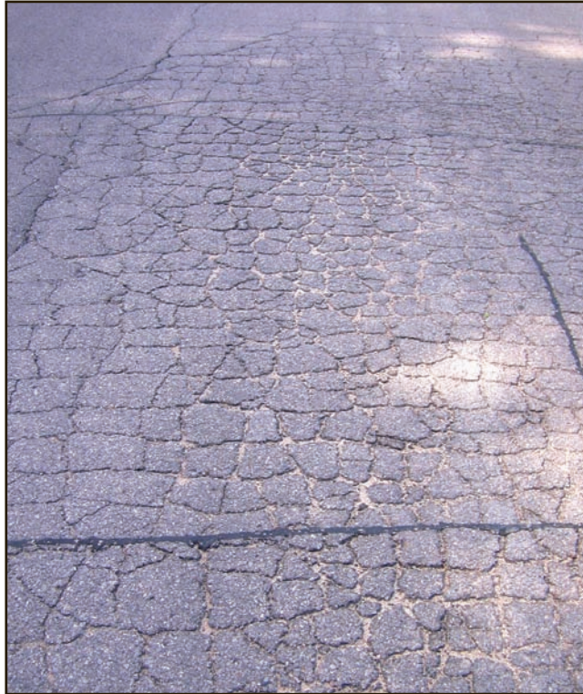
Figure 8. High alligator cracking is a network of cracks that have formed and grown into blocks. Areas where dense cracks have formed pump when loaded.
