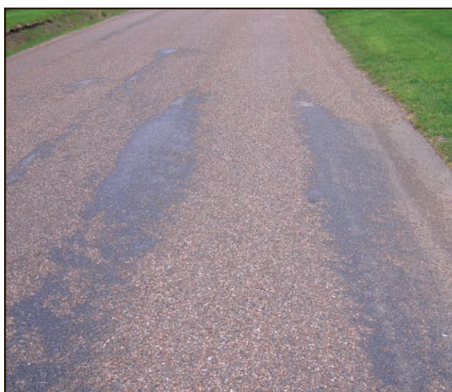
Figure 25. High severity raveling of a seal coat.
