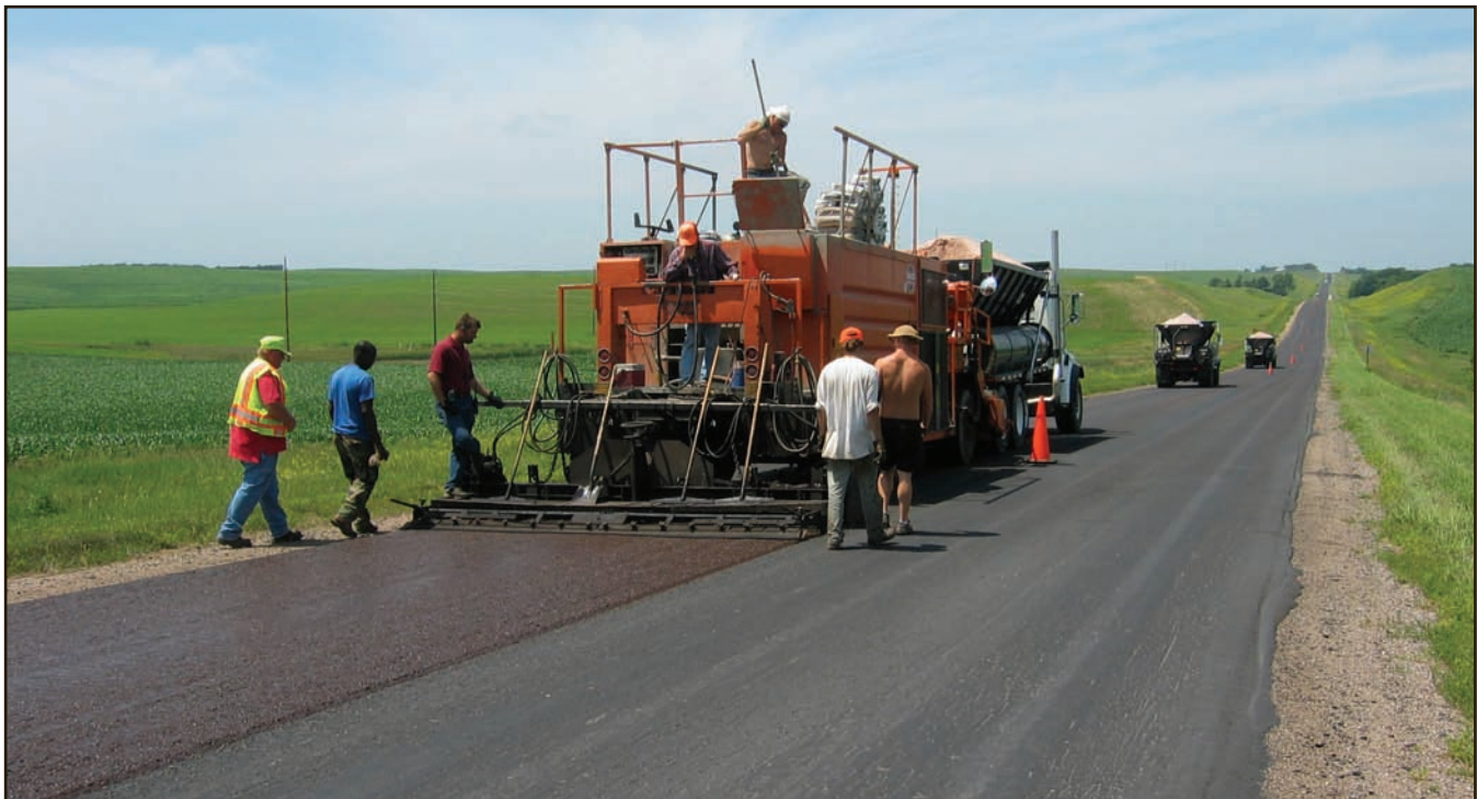
Figure 30. Micro-surfacing application.
