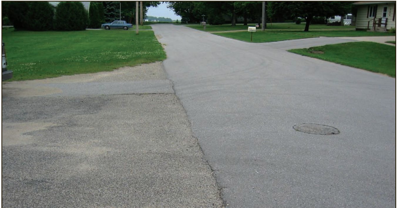
Figure 32. Smooth seal overlay on existing seal coat road.
