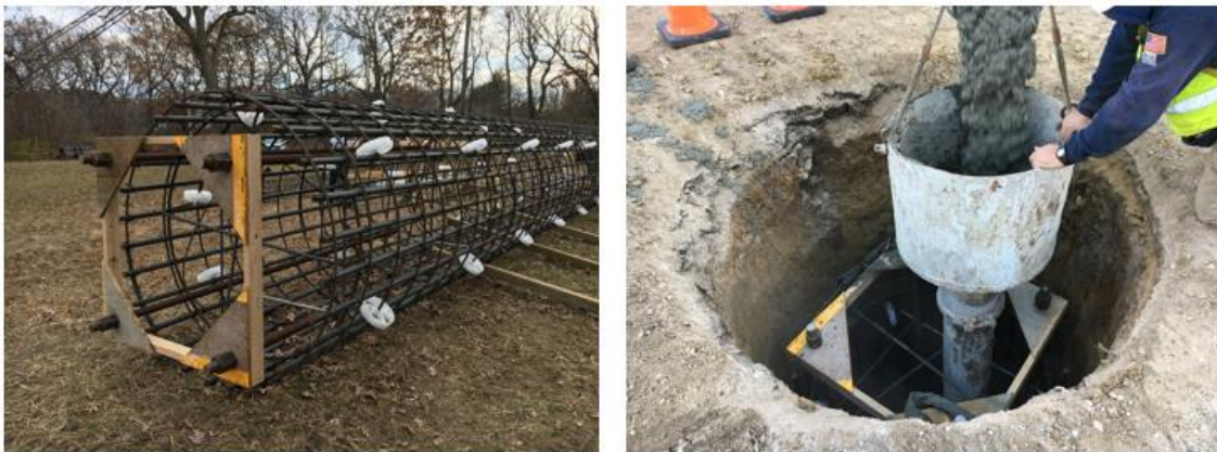
Figure 5.27. Construction of drilled shaft
