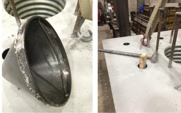
Figure 5.13. Taking out reusable reducers
