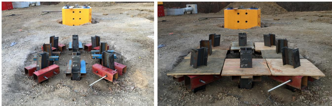
Figure 5.17. Friction collars and plywood seal-pads
