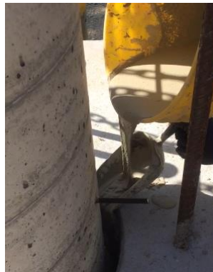
Figure 5.19. Grout pouring
