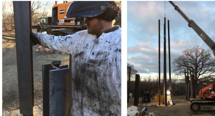
Figure 5.16. Weld-splicing piles
