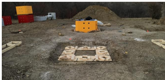
Figure 5.15. Driven pile template
