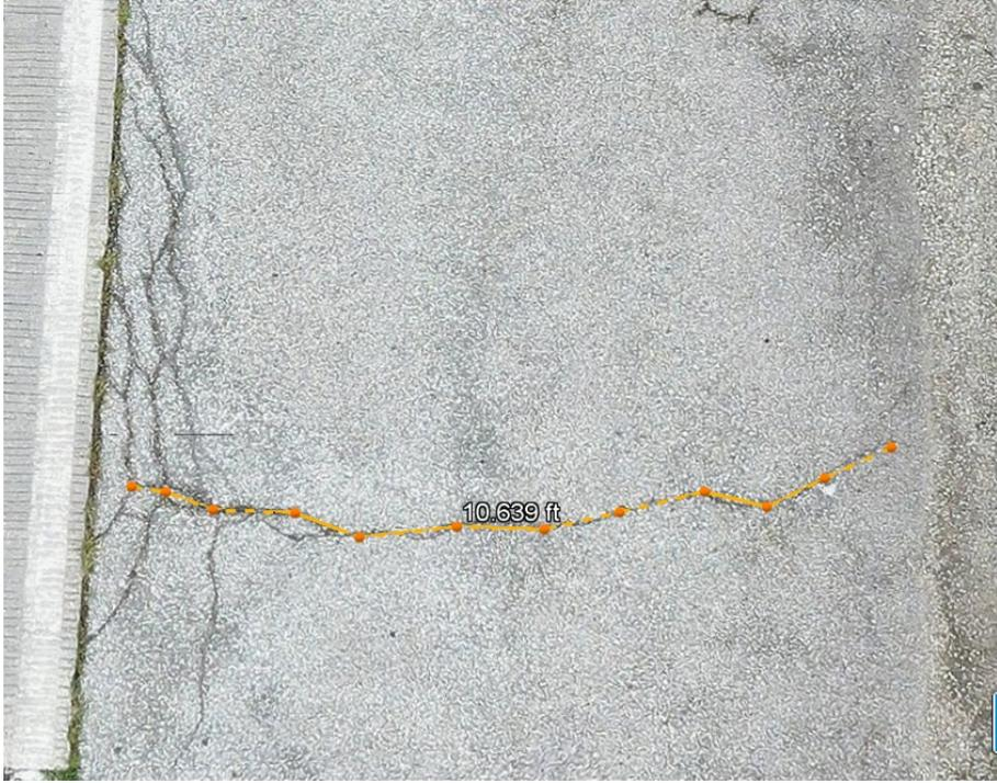
**Figure 3.9. Measurement of the length of a crack**
