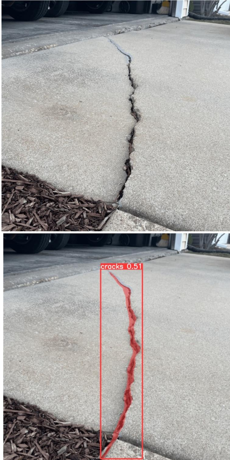
**Figure 4.17. Result of concrete crack detection before and after an image is uploaded to the model**
