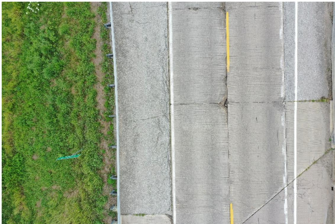
**Figure 3.3. Example of an image captured by Mavic 2 Pro drone from a 50 ft distance**
