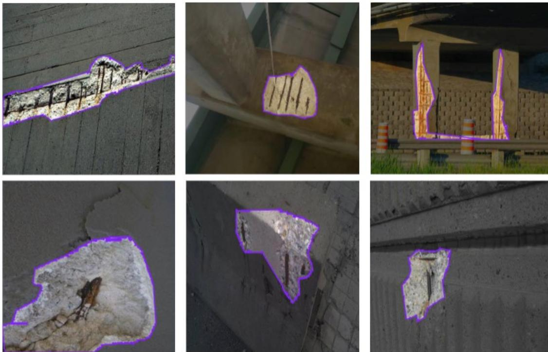
**Figure 4.10. Annotated images for concrete spalling**
