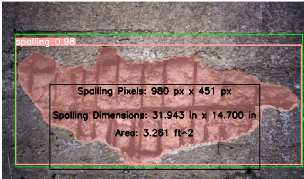
**Figure 4.24. Result of concrete spalling quantification**
