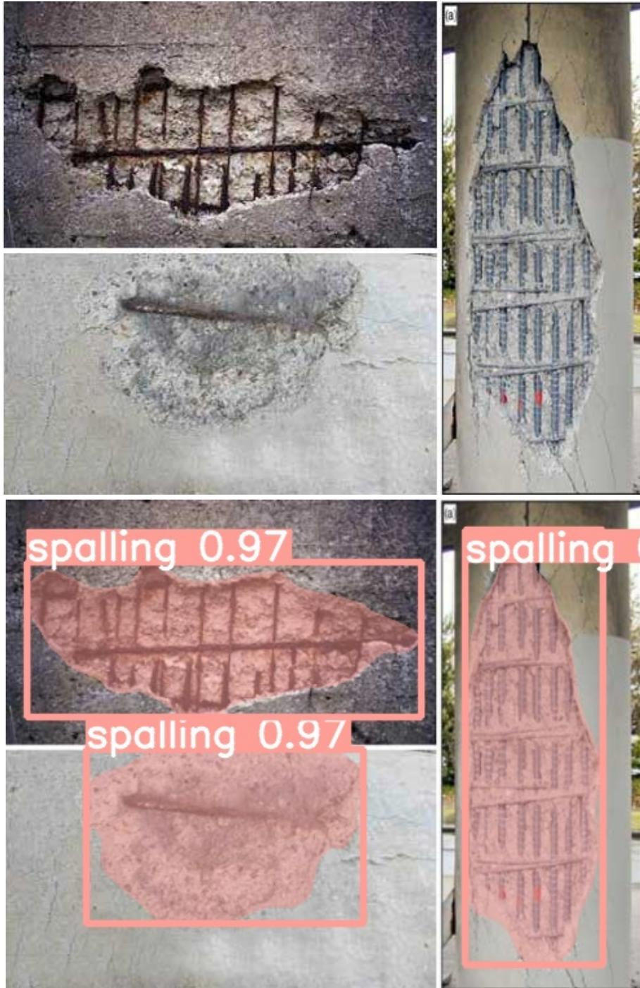
**Figure 4.19. Result of concrete spalling detection before and after an image is uploaded to the model (testing for the detection of multiple damage types in different backgrounds)**
