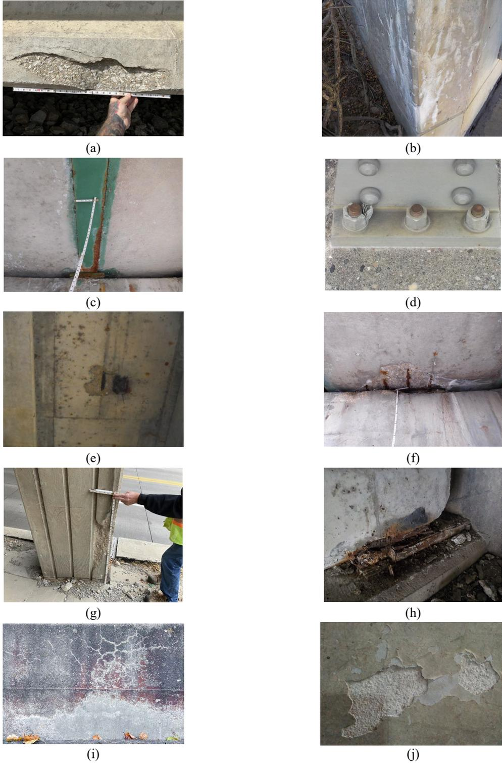
**Figure 2.2. Examples of other types of damage observed in bridge components: (a) concrete spalling, (b) efflorescence, (c) girder corrosion, (d) galvanic corrosion in bolts, (e) rebar exposure, (f) rebar corrosion, (g) concrete column spalling, (h) bed corrosion, (i) concrete discoloration, and (j) concrete delamination**
