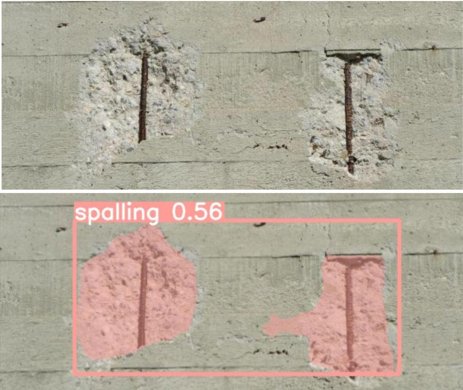
**Figure 4.18. Result of concrete spalling detection before and after an image is uploaded to the model (testing for the detection of multiple damage types in one image)**
