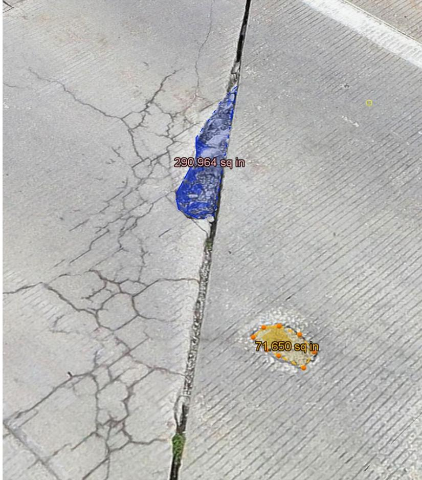
**Figure 3.10. Measurement of the area of a defect**
