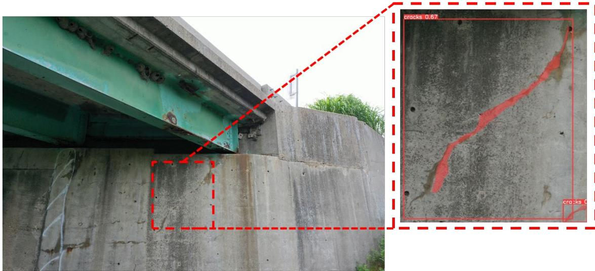
**Figure 4.20. Result of concrete crack detection before and after an image is uploaded to the model (image from case study bridge)**
