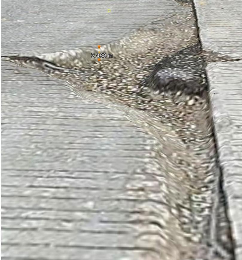
**Figure 3.8. Measurement of the depth of a pothole**
