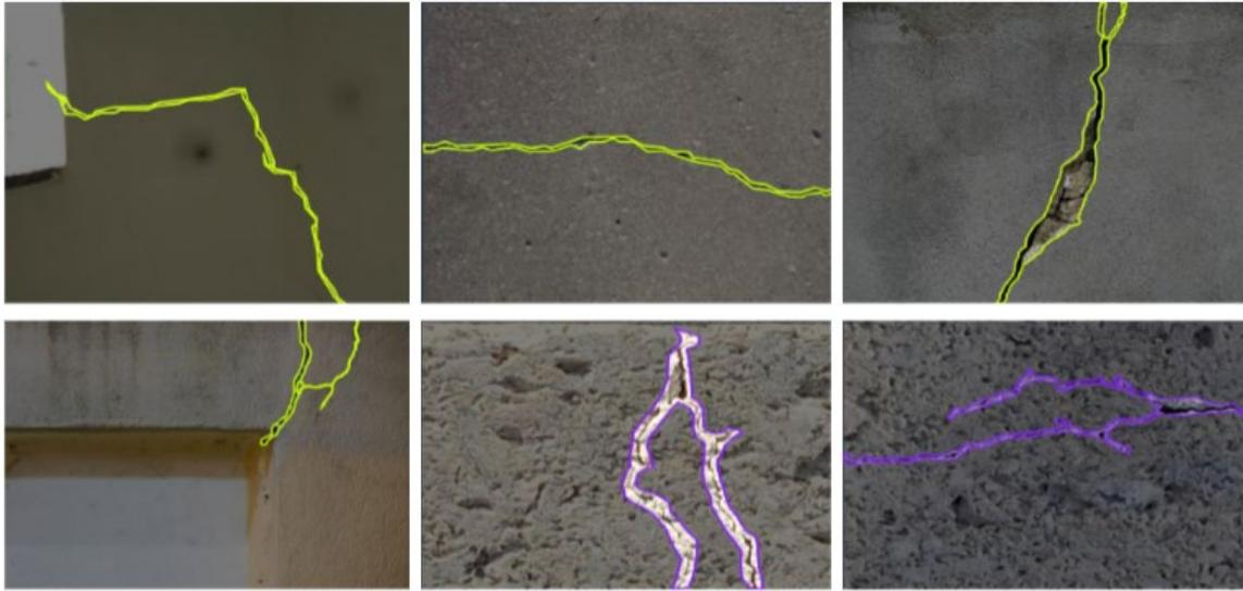
**Figure 4.9. Annotated images for cracks in concrete**
