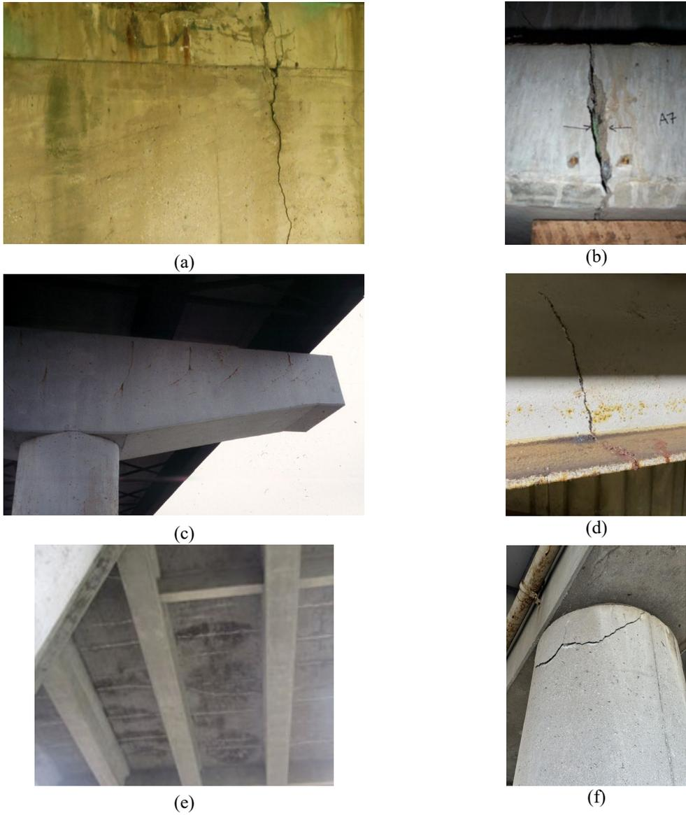
**Figure 2.1. Examples of cracks in bridge components: (a) abutment, (b) concrete girder, (c) pier, (d) steel girder, (e) deck, and (f) column**
