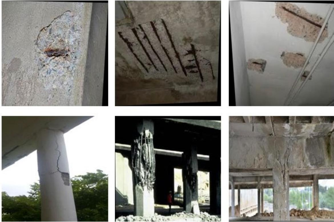
**Figure 4.8. Pre-annotated images for concrete spalling (various backgrounds and distances)**
