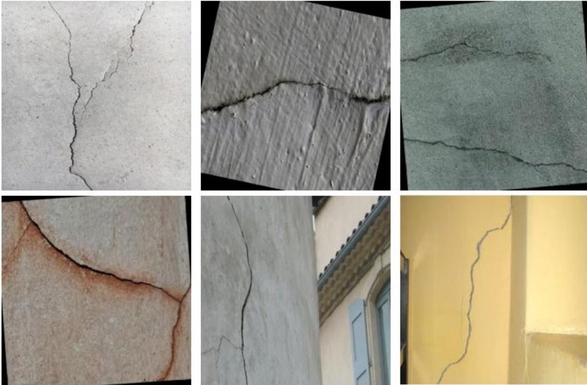
**Figure 4.7. Pre-annotated images for cracks in concrete (various backgrounds and distances)**
