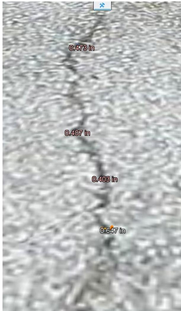
**Figure 3.11. Measurement of the width of a crack**
