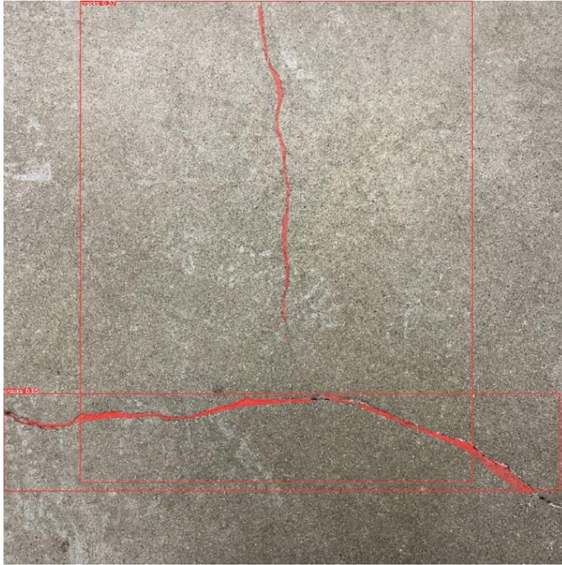
**Figure 4.16. Result of concrete crack detection after the image is uploaded to the model**
