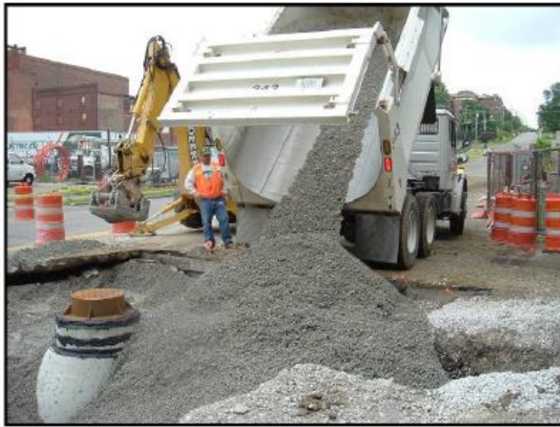
Figure 9D-1.02: Large Lift Thicknesses Used in Utility Cut Trench Backfill Material Placement
