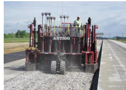
Rubblizing - Photo courtesy of Antigo Construction
