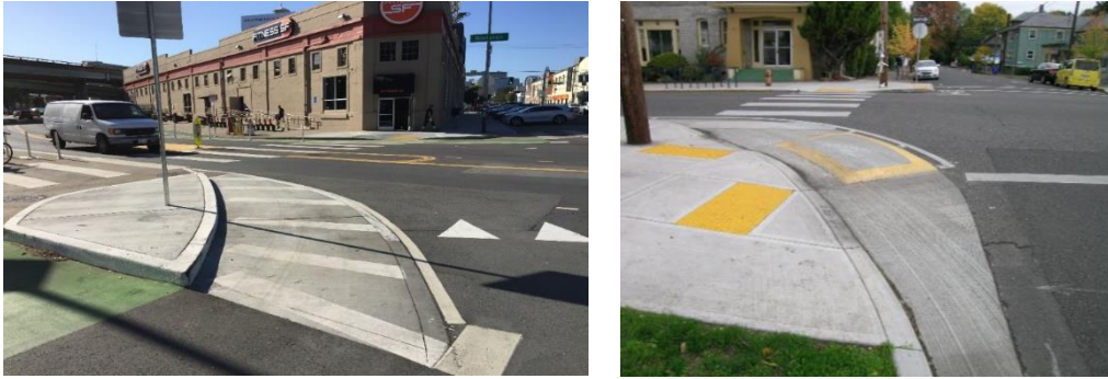
Figure 5M-1.04: Truck Apron with Concrete and Pavement Markings (left) and Truck Pillow (right)
