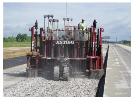
Rubblizing - Photo courtesy of Antigo Construction
