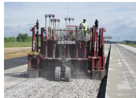
Rubblizing - Photo courtesy of Antigo Construction
