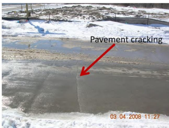
Figure 14B-2.07: Pavement Cracking Caused by HDD Installation
