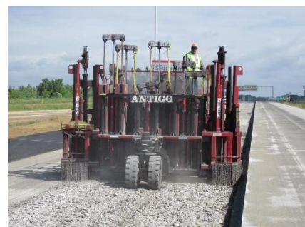
Rubblizing - Photo courtesy of Antigo Construction
