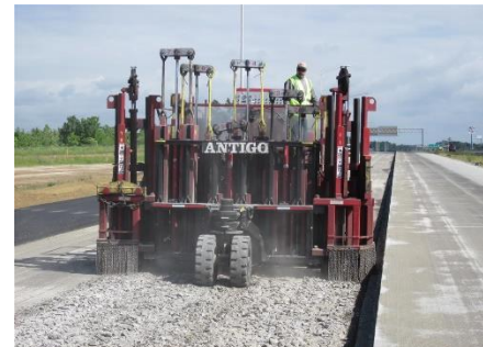
Rubblizing - Photo courtesy of Antigo Construction
