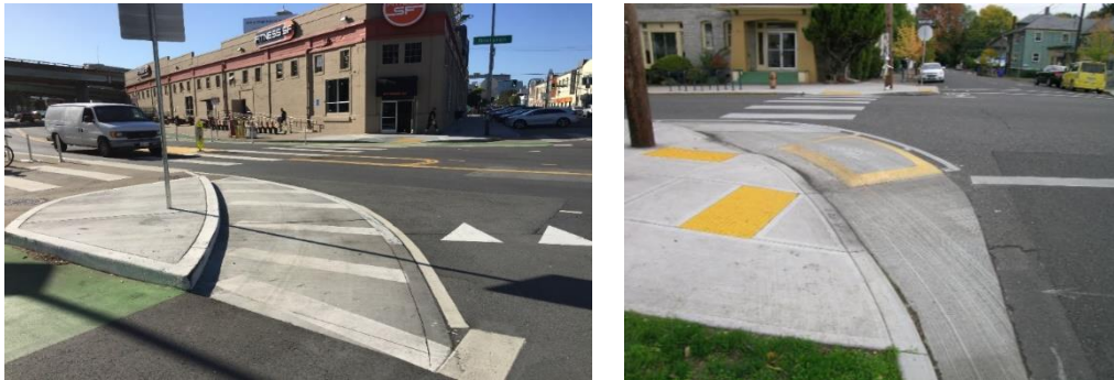
Figure 5M-1.04: Truck Apron with Concrete and Pavement Markings (left) and Truck Pillow (right)
