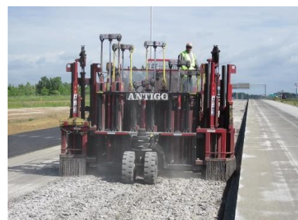
Rubblizing - Photo courtesy of Antigo Construction
